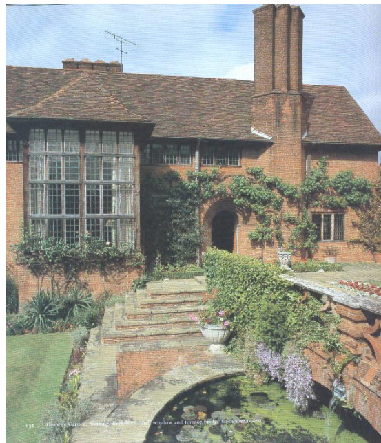
grote lichtopening in traditioneel gebouw – arch. Edwin Lutyens Deanery Garden, Sonning, Berkshire, 1902
